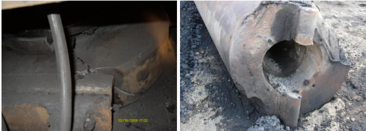
Figure 1. EKG-10 shovel's kingpin fracture under operational loadings
